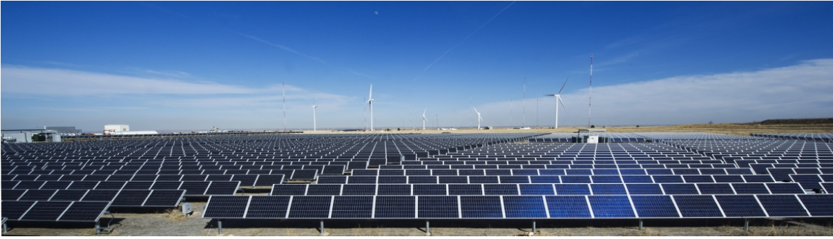
Photovoltaic panels (source: U.S. Dept. of Energy)
